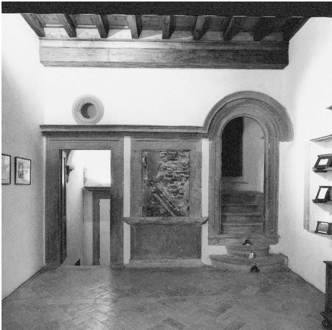
Well-staircase probably once part of the Torre de' Pulci, discovered and restored during work carried out after 1993
